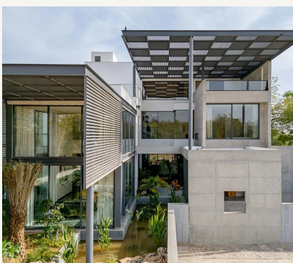
MUMBAI • 2024 • THE LOUVRE HOUSE
